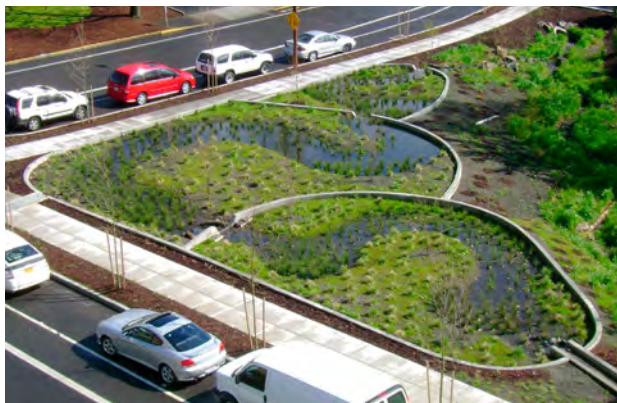
Headwaters at Tryon Creek, SW Portland. The rounded and stepped design of these infiltration planters are molded to the specific conditions of the site. The concrete walls are a creative interpretation of check dams that are used to convey water across flat surfaces over steep topography.
