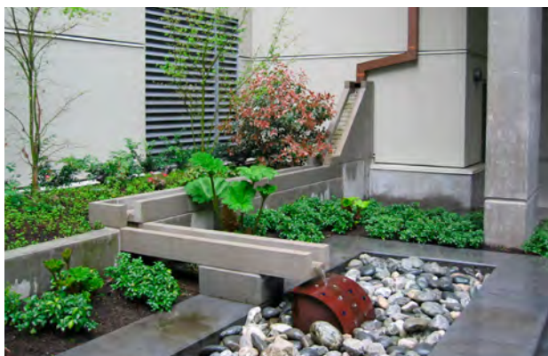
10th @ Hoyt, Portland. The design of this urban courtyard is inspired by Persian gardens. Downspouts convey stormwater from the surrounding rooftops into a series of channels and colorful fountains.
