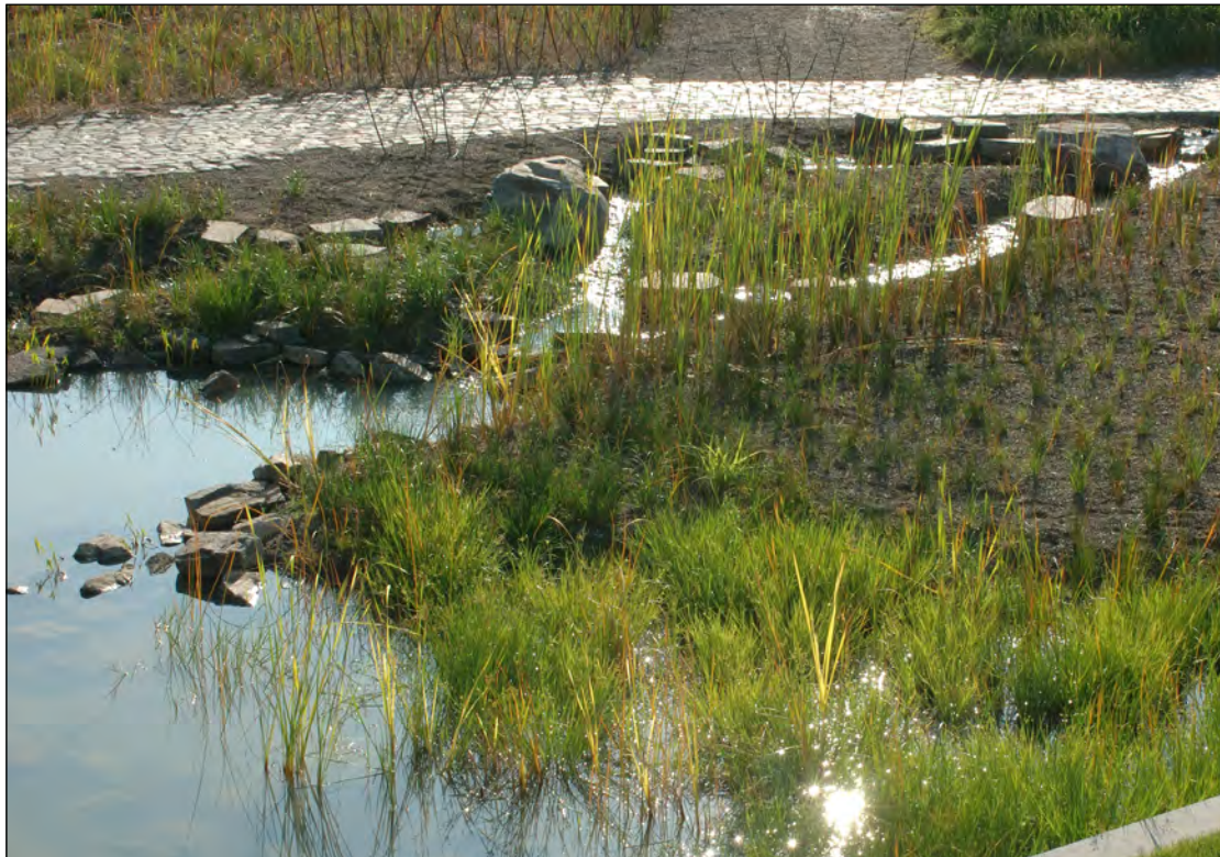
Tanner Springs Park, Portland. Stormwater from surrounding impermeable surfaces is conveyed and recirculated through a constructed wetland and filter strip to be cleansed and aerated. The filter strip and wetland edge is planted with a variety of native plants based on their suitability to the different planting conditions.
