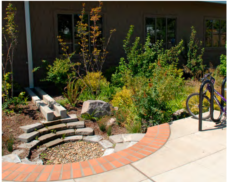
Estacada Library. Stormwater is conveyed from the rooftop to an infiltration basin. As the basin fills with water, it overflows into a connected series of swales and additional infiltration basins that convey stormwater around the library.
