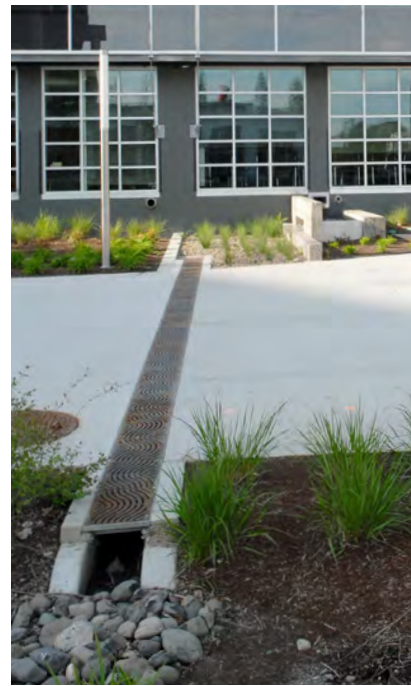
RiverEast Center, Portland. Stormwater from the rooftop is conveyed by a downspout into a sculptural basin made with reclaimed concrete from the retrofit of the building. The basin detains and slows runoff before it flows into a series of adjacent rain gardens, grated runnels and swales.
