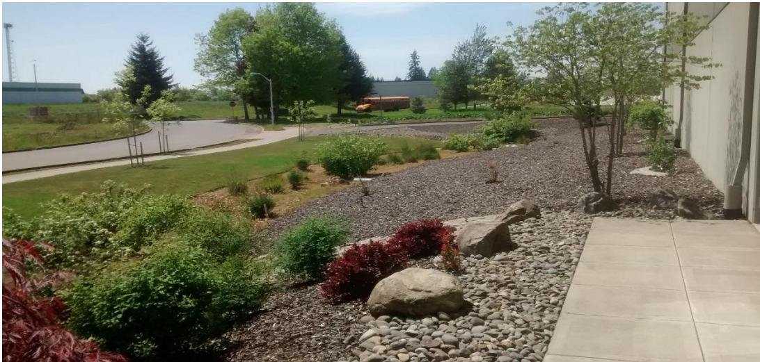
Stormwater Bio-swale Located at Dragonberry Produce, Inc.
