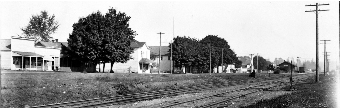
SC 017, Main Street (NW 1st Ave), 1909. Main Street (now NW 1st Avenue), west of the railroad depot had numerous business buildings in Canby's early days. Pictured from left are a furniture store, the William Knight building (1891) on the Fir Street corner, the first city hall, early post office location, and other buildings east of N. Grant Street. Canby Historical Society.
