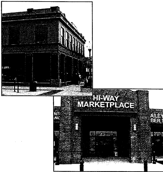
Figure 23 These buildings in the commercial core illustrate desired design features in
