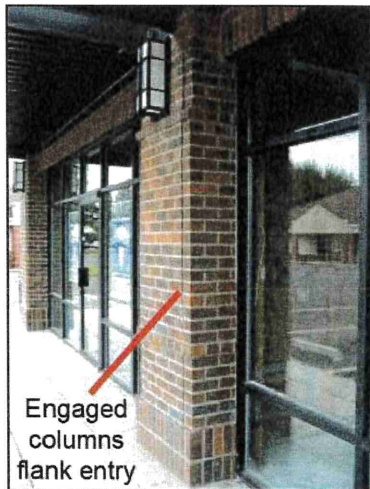
Figure 43 Entry flanked by engaged columns and lighting
