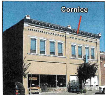
Figure 58 Cornice used on flat roof
