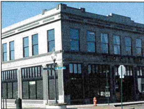
Figure 19 Design details such as a recessed entry, columns and decorative transom windows help articulate the ground floor and distinguish it from the upper floors
