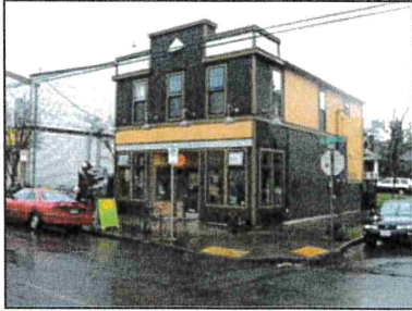
Figure 32 Top of building features a parapet
