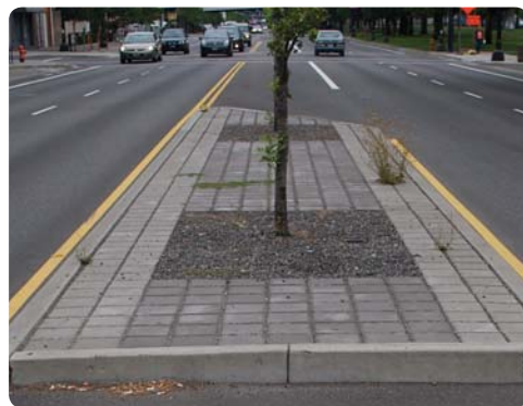
Paved median example
