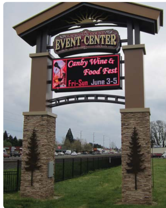
Event Center stonework
