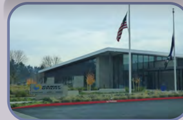
Canby Utility's new office is located at 1265 NE 3rd Ave
