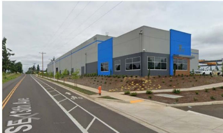
Heavy Manufacturing (Lampros Steel)
