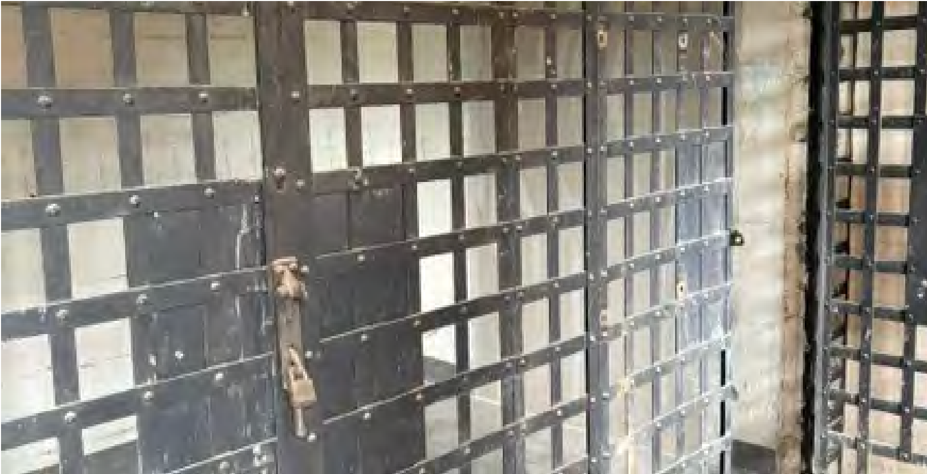
Jail cell doors – Holly Street City Hall
