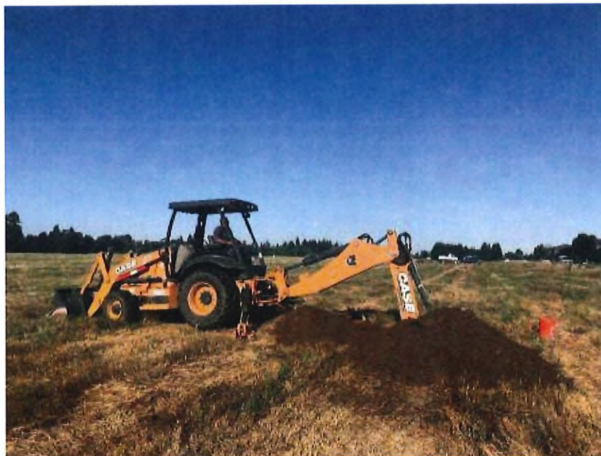
Backhoe Test Pits
