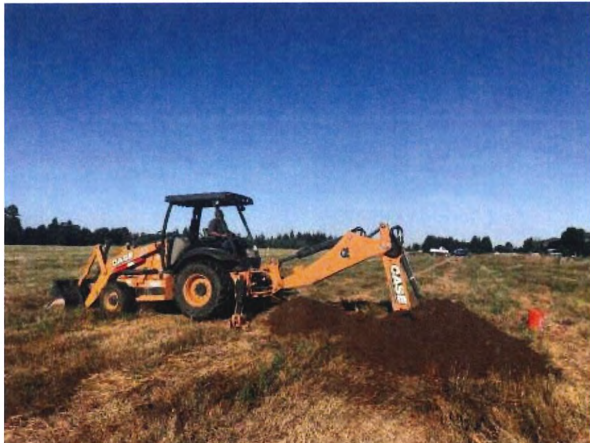
Backhoe Test Pits
