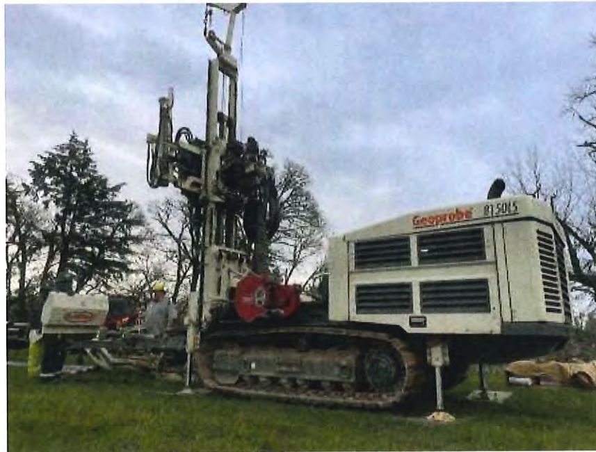
Sonic Drill Rig Soil Borings
