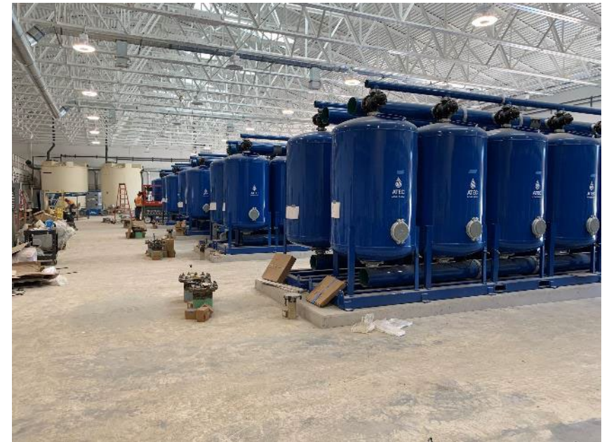
Manganese Filter Installation at Rockwood Water PUD, Gresham, OR
