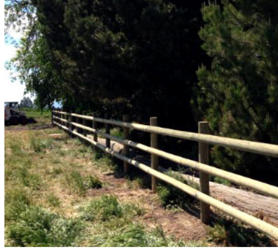
Figure 14. Example of Context-Sensitive Fencing Using Natural Materials
